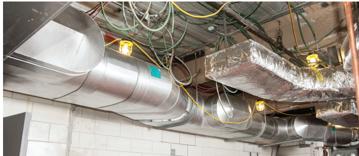
SlimVent's flat oval design makes it ideal for grease duct installations where round products do not meet overhead clearances, providing up to 28% space savings.
